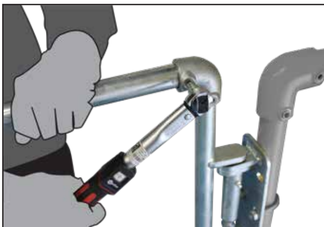
I. Carefully re-position the gate top and bottom tubes into the cast fittings. Ensure the striking plate is on the correct side of the Support Leg/Structure. Use a spirit level to ensure the gate is level. Tighten the cast fittings grub screws using a hex head socket. Using the torque wrench ensure the castings are torqued to 39Nm.
