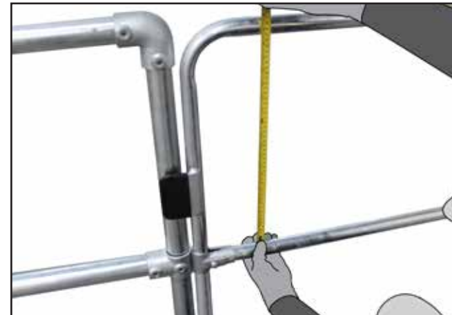
Q. Use a measuring tape to ensure the gap between top rail and mid rail is no more than 470mm. Adjust if necessary.
