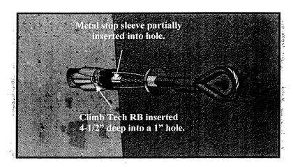
Only use industrial grade rotary hammer drills and drill bits.
